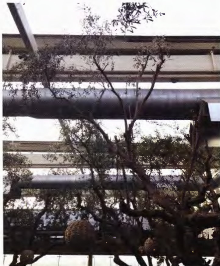
Some of the dieback was near the HVAC vents. Could the vents be the cause of the dieback?
