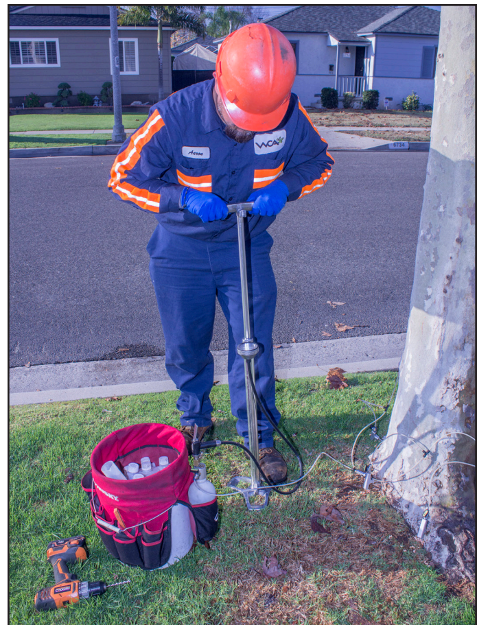
Soil injection treatment application. Photo by Donald R. Hodel.
