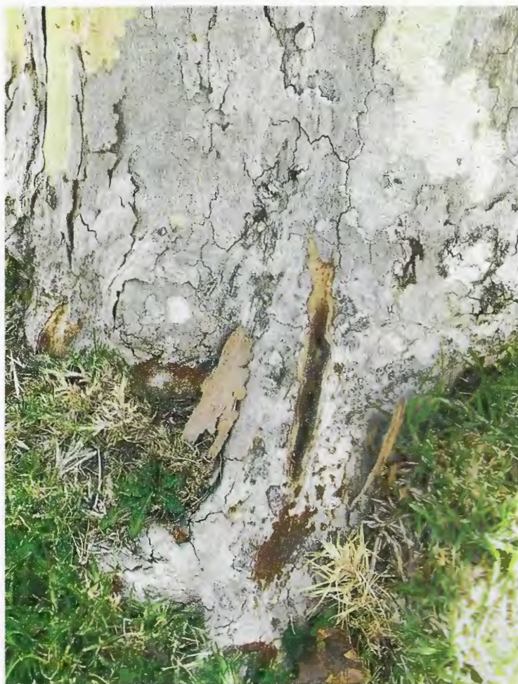
Wounding on a buttress root caused by a trunk injection.
