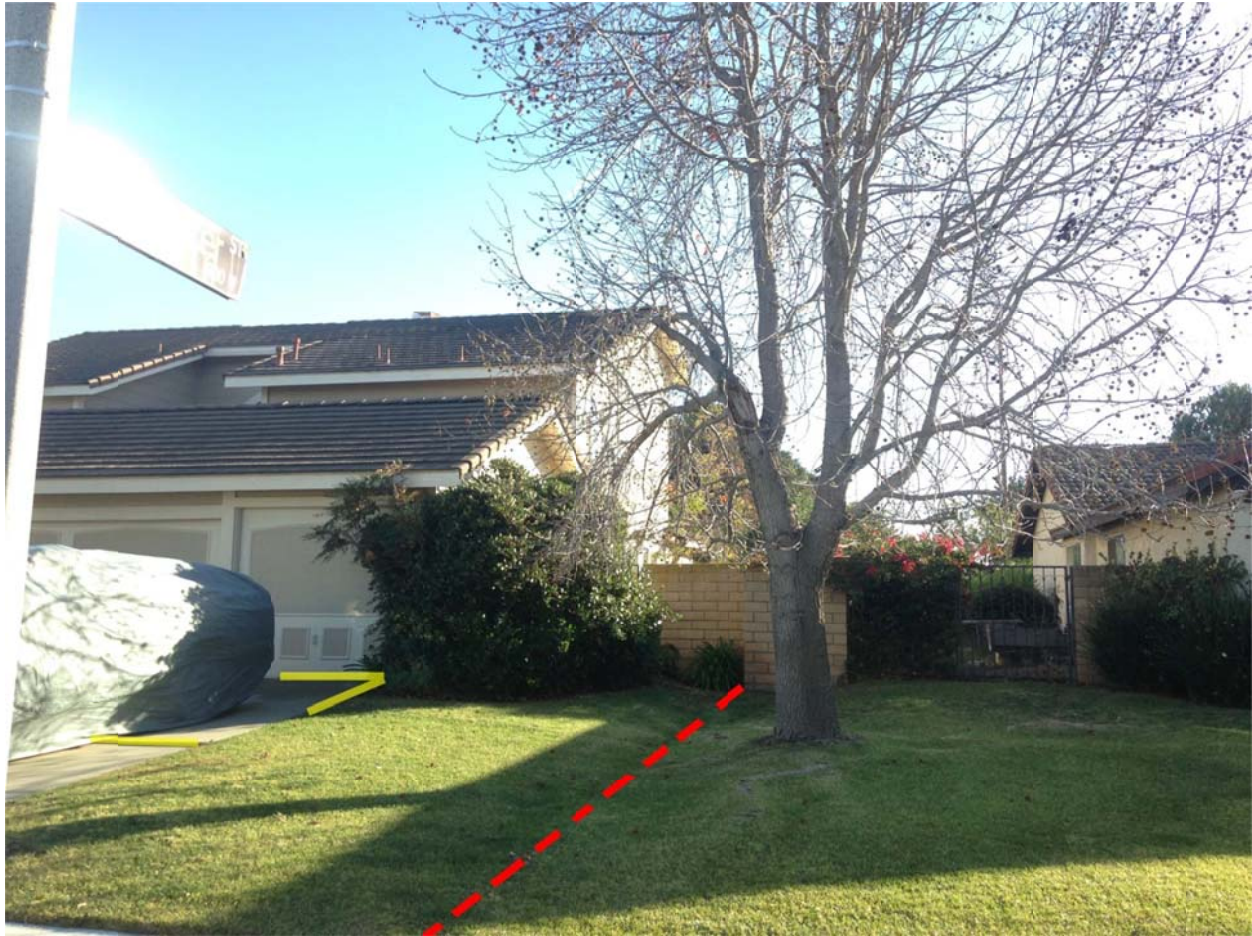
Figure 2: Looking south at the subject Liquidambar tree. The driveway displacement is highlighted in yellow. The Raphiolepis shrub is next to the garage. It is not likely that this shrub caused the driveway displacement. The displacement in the middle of the driveway (far left) was approximately 1.5 inches, and the displacement nearest to the garage was approximately 1 inch.
