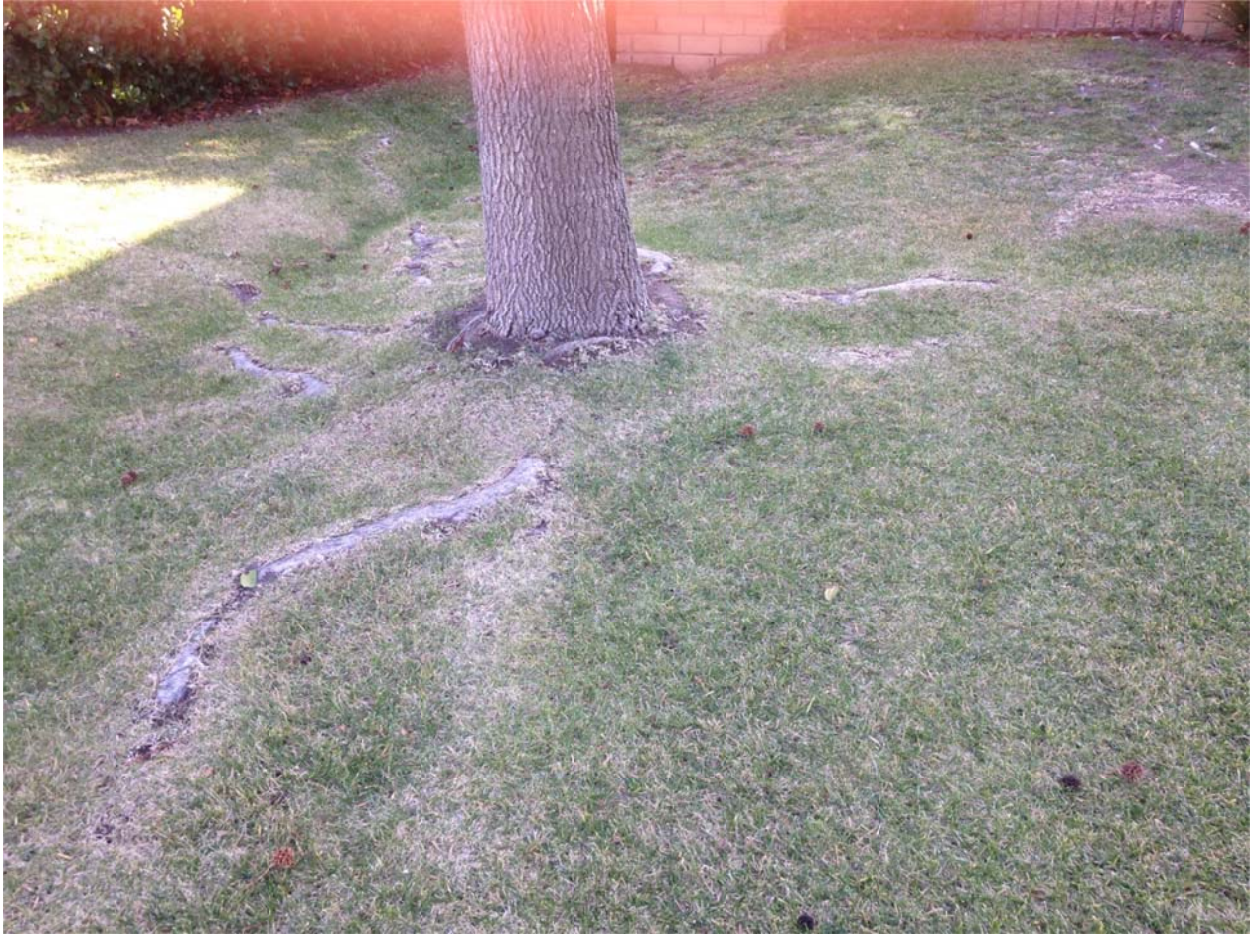
Figure 6: Surface roots of the subject Liquidambar tree. These roots became apparent above the soil level in the last 4 years according to the client.
